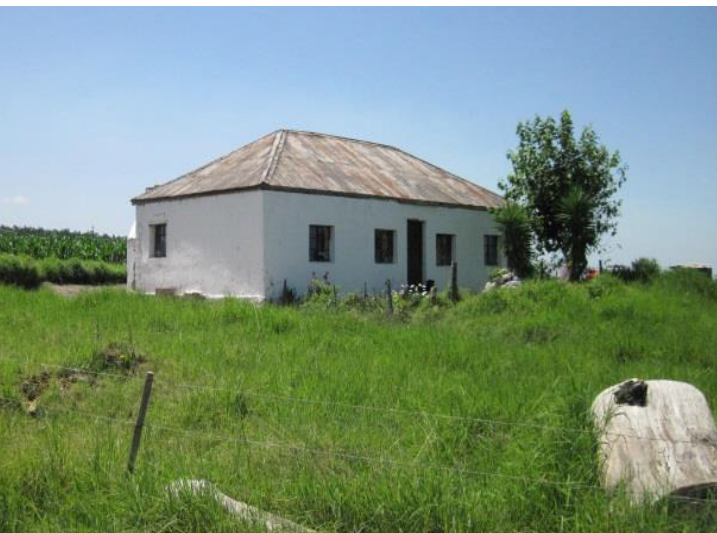
Figure 18: Cottage located at proposed intervention area 1
